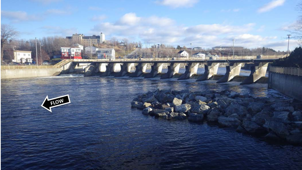
Figure 3. Mathieu-D'Amours Dam viewed from downstream (MDDELCC).
