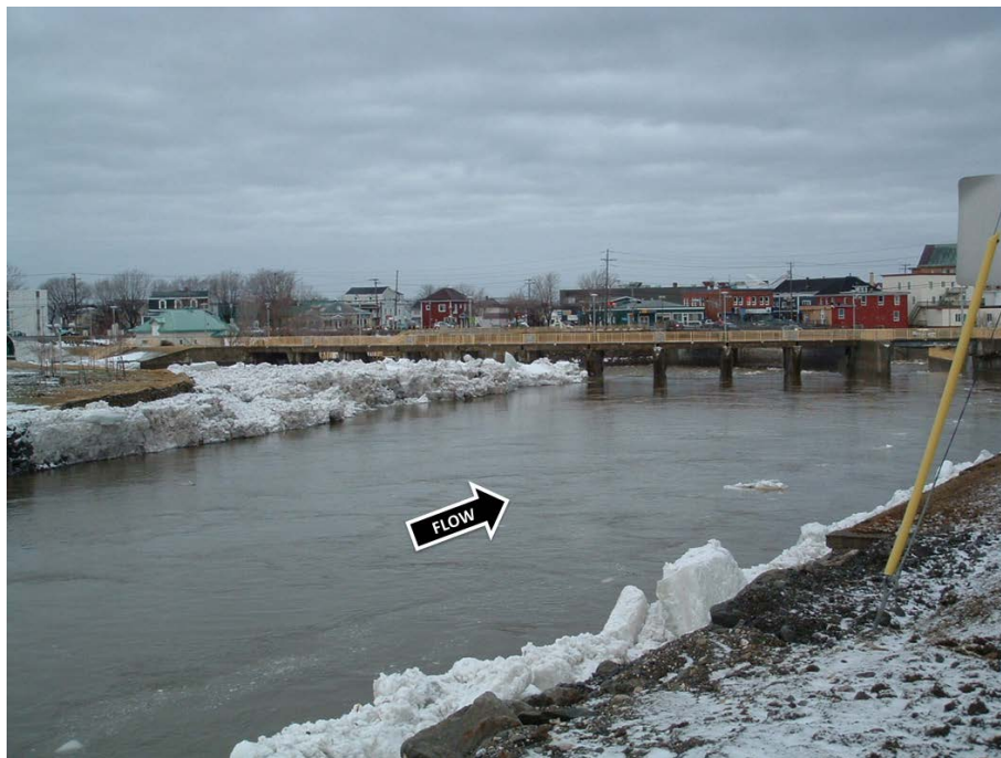
Figure 4. Ice remains upstream of the dam after breakup on April 6, 2009 (MDDELCC).
