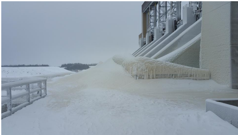
Figure 3. Buildup of several metres of ice on a deck from the spray of a spillway operated during the winter. (Photo: Manitoba Hydro)
