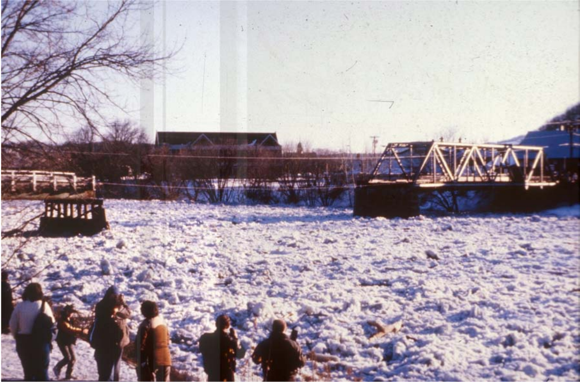
Figure 2. Failure of the White River Bridge, 27 Jan. 1990 as a result of ice jam induced scour around piers.
