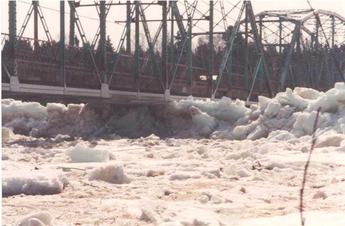
Fig. 1. Ice striking the bottom chords of the Quarryville Bridge on the Southwest Miramichi River, New Brunswick, April 15, 1994.
