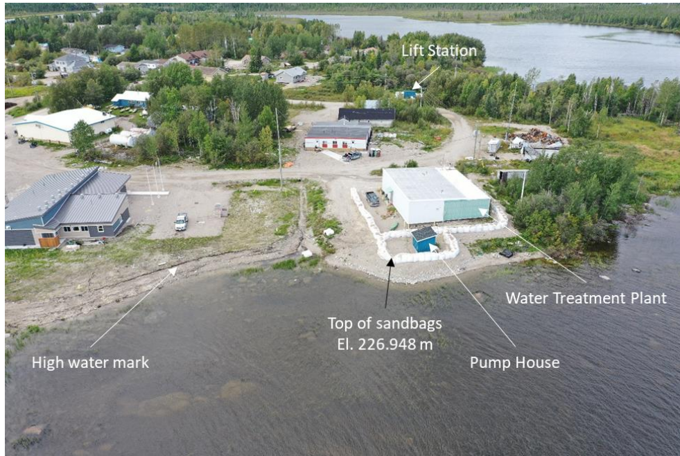
Figure 10. Sandbag dikes constructed to protect water treatment facility and pump station
