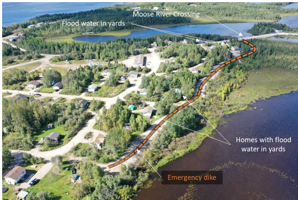
Figure 11. Emergency dike constructed to protect homes on Michikan Lake
