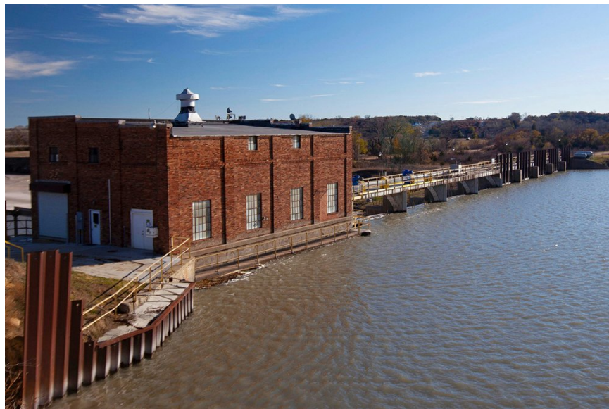
Figure 3. Photo of Spencer Dam powerhouse and spillway operating in November 2013 (Source: NPPD)
