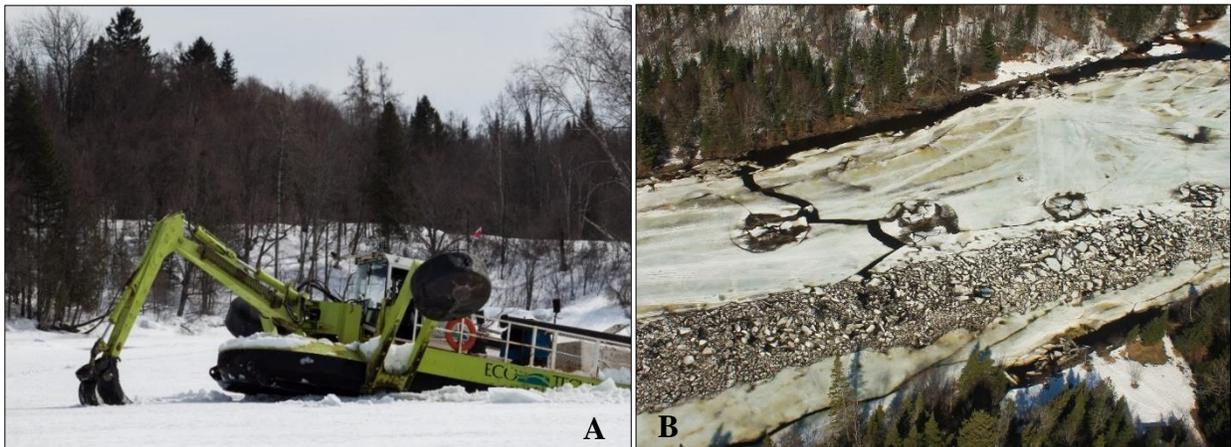
Figure 2. (A) Amphibex at work at km 0.3 on the St. Anne River and (B) channel made by the Amphibex at km 1.3, 8 days after the end of the ice weakening measure. The ice cover depicted presents several signs of advanced deterioration (cracks and open spots) even on the side of the channel. Of interest in the picture is the presence of artificial islands (old rafting boxes).
