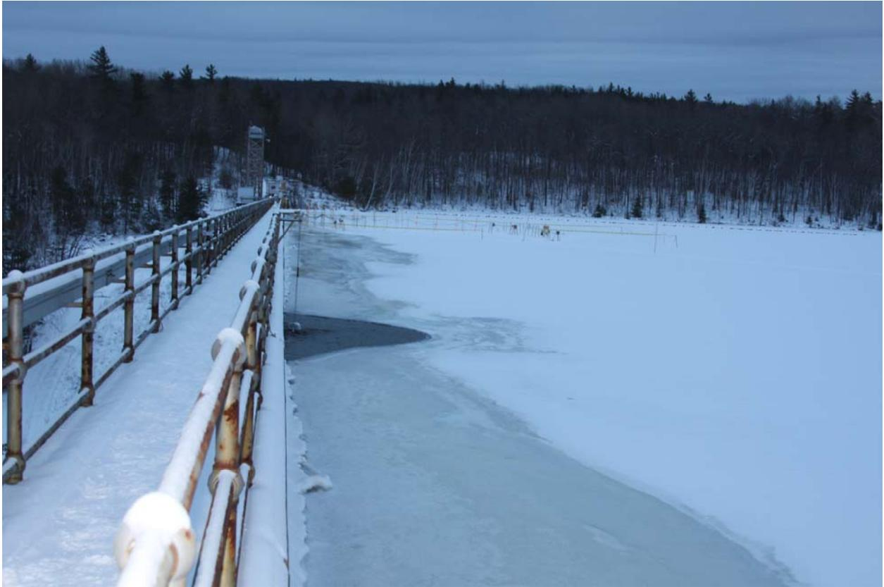
Figure 1. Dam at Barrett Chute. Note flooding near dam face; artificially open section to measure levels; and instrumented section near center. Photo taken from left bank (Morse).
