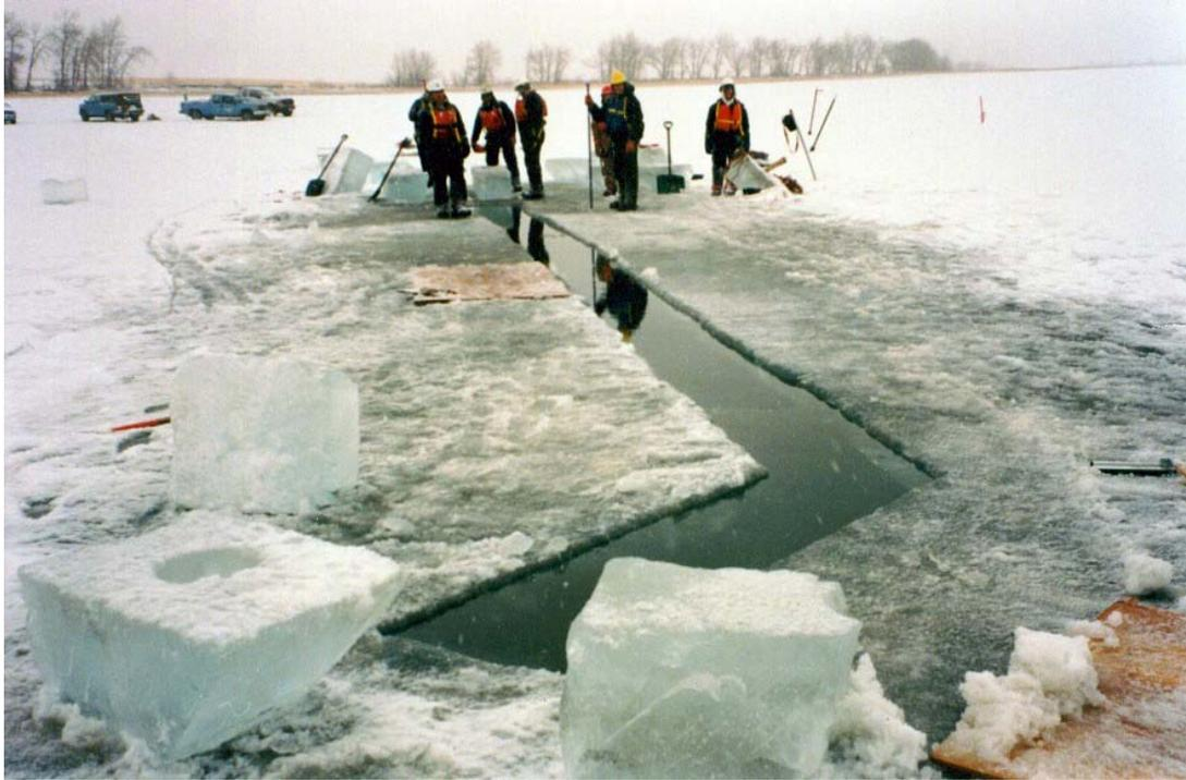
Figure 1. An ice slot designed to intercept an oil spill under a river ice cover.
