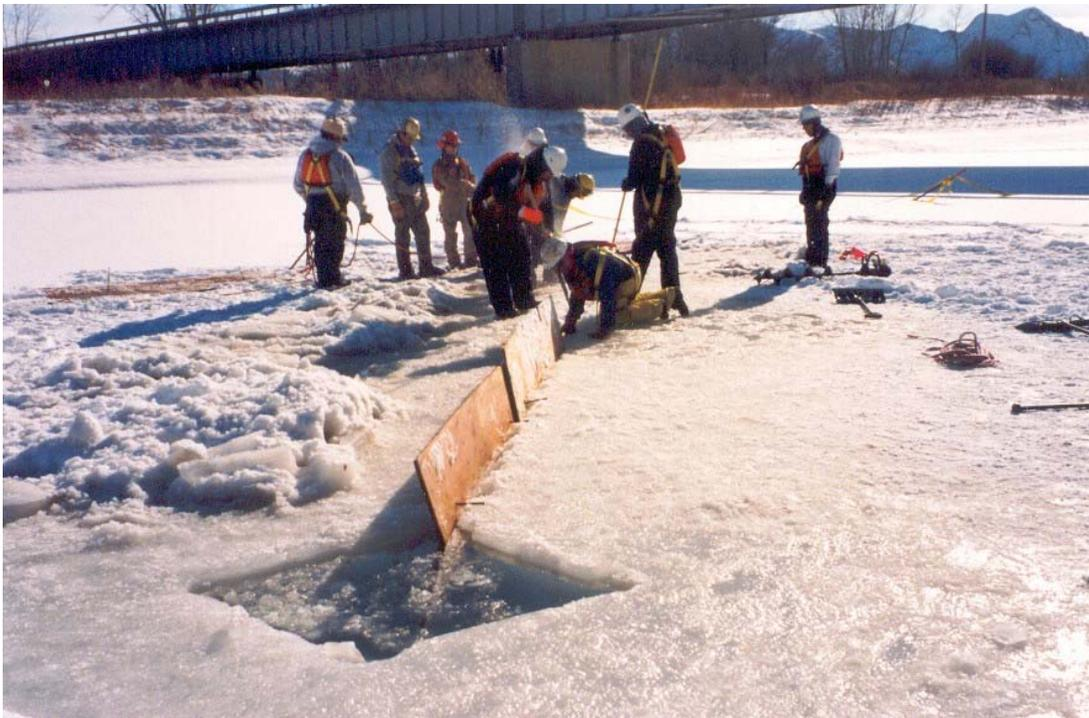
Figure 2. A diversionary barrier made of plywood sheets and a sump to contain an oil spill underneath a river ice cover. (Photo source: Dowcar Environmental Management, Inc.)
