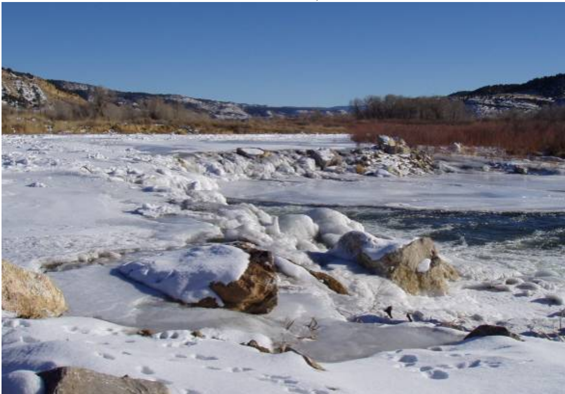
Fig. 2. Freezeup ice jam on the White River in northwestern Colorado caused by the heightening a rock diversion weir.
