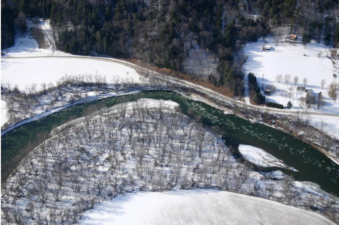
Fig. 1. Rock vanes deflecting flow and frazil ice away from a bank in the Winooski River near Williston, VT.
