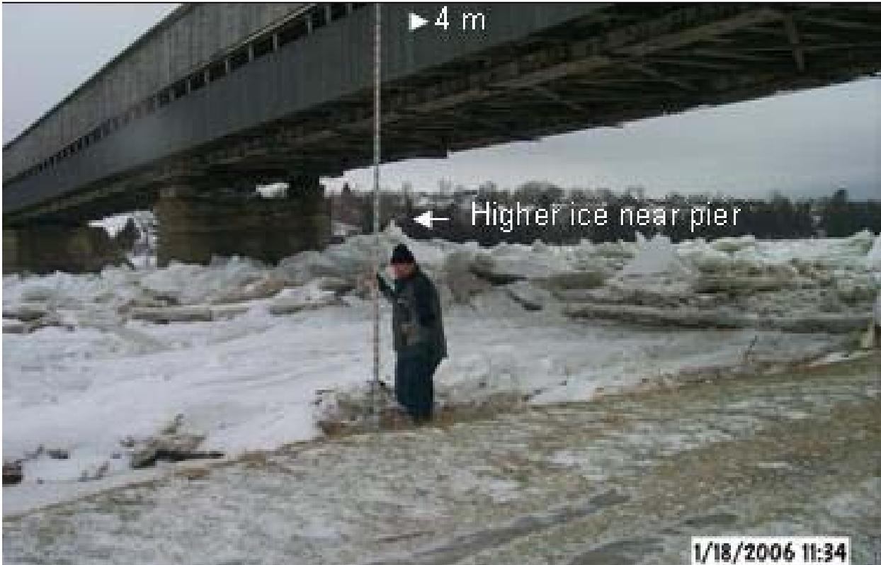
Figure 4. Looking across and slightly upstream from left bank at the Hartland Covered bridge, the photograph shows that the bridge superstructure was generally over 3 m above the top of the ice jam. Photo was taken by T. Doyle, Hydro-Com Technologies.
