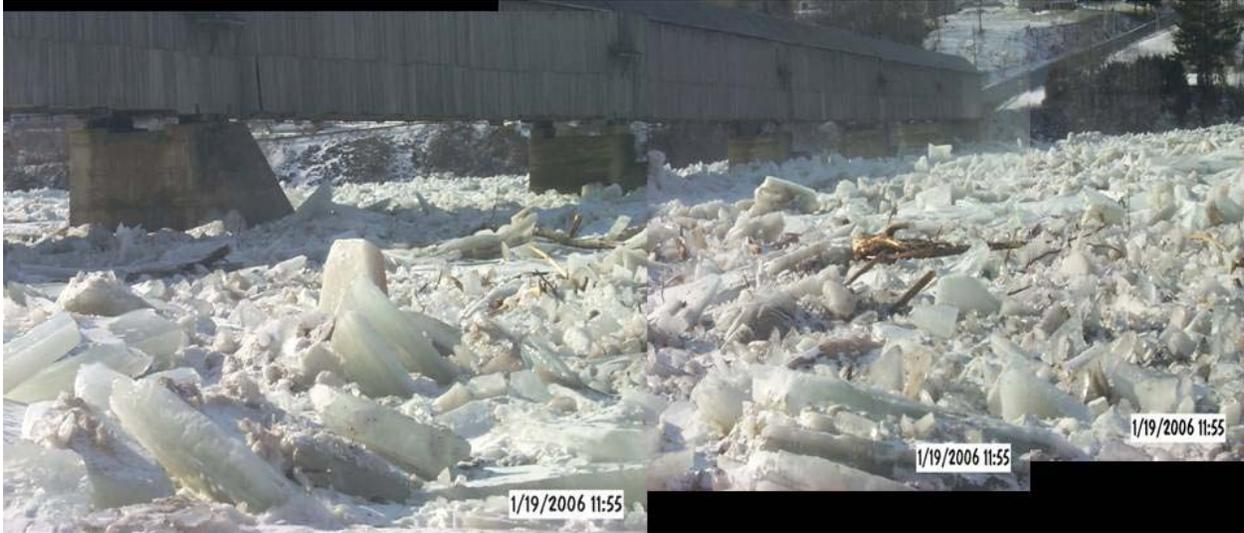
Figure 3. Photo mosaic looking downstream from the left bank towards the piers of the Hartland Covered bridge shows the rubble ice and debris on the upstream side of the bridge. Generally, the middle portion of the ice jam, from the Hartland Covered bridge to the Hugh John Fleming bridge, contained larger ice rubble generally thicker than 15 cm.
