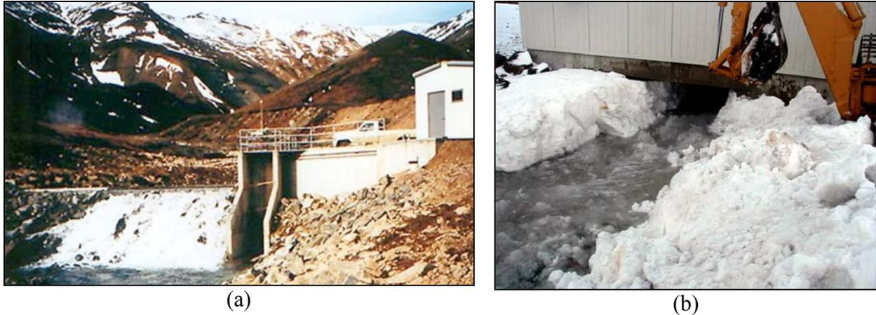
*Figure 9. King Cove micro-hydro plant, Alaska (a); excavation of frazil from the plant's small tailrace channel (b) (Photos courtesy of King Cove Hydro)*
