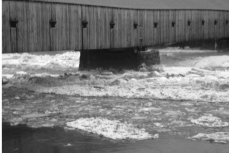
*Fig. 14 -- Thick, rafted brash ice and dispersed brash ice in largely open water are both visible near the Cornish-Windsor bridge. These conditions occurred later in the breakup sequence as ice concentration was diminishing. View is from the left bank looking across and downstream.*
