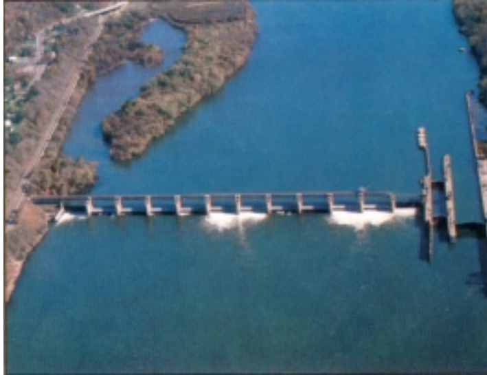
Figure 1. Photo of the Montgomery Locks & Dam (looking upstream)
