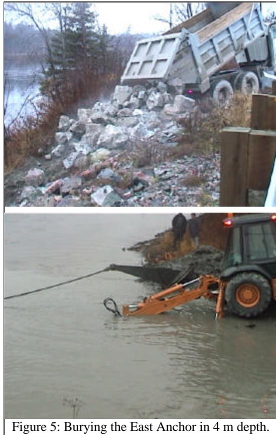
Figure 5: Burying the East Anchor in 4 m depth.
