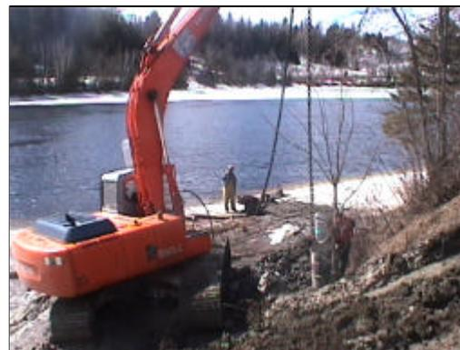
Figure 11: Deployment of the chain inside the concrete filled 15 cm casing.
